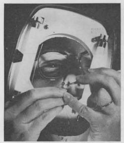
THIS TINY TOROIDAL transformer was carefully wound by hand in Sandia's Transformer Section. It's inspected here under an illuminated magnifier by Helen Agats, who uses tweezers to separate hairlike lead
